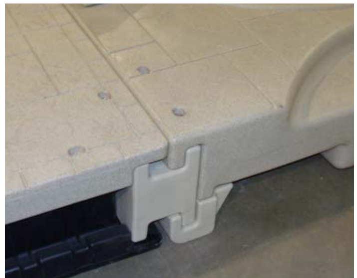
H-Beam in place
